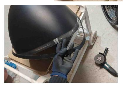
Cut it carefully with a thin disk. Be careful this releases a lot of dust.
