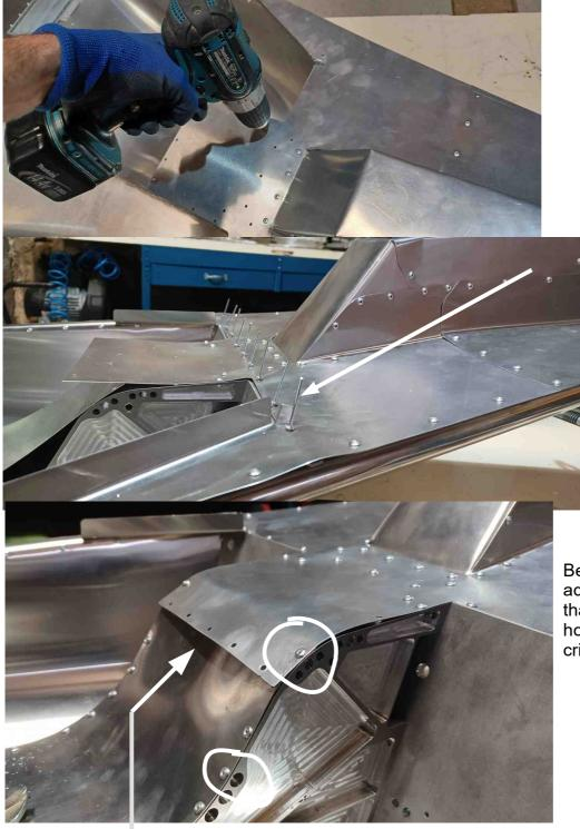
Finish riveting the T14 tubes then continue to rivet the sheet metal onto the N10 rib, while drilling, respect the angle of the rib.
