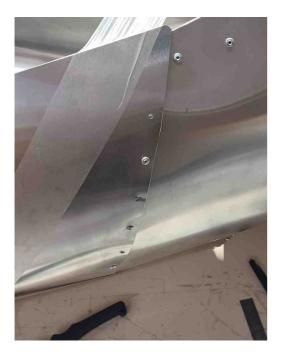
Complete the drilling and install the rivets.
