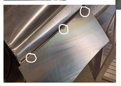
Fix 2 or 3 rivets and check if by bending the sheet, the distribution is still balanced to the right and left
